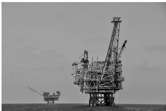
Figure 14.2 Tamar gas field production platform in the Mediterranean Sea. Photo by Ilan Nisim.
